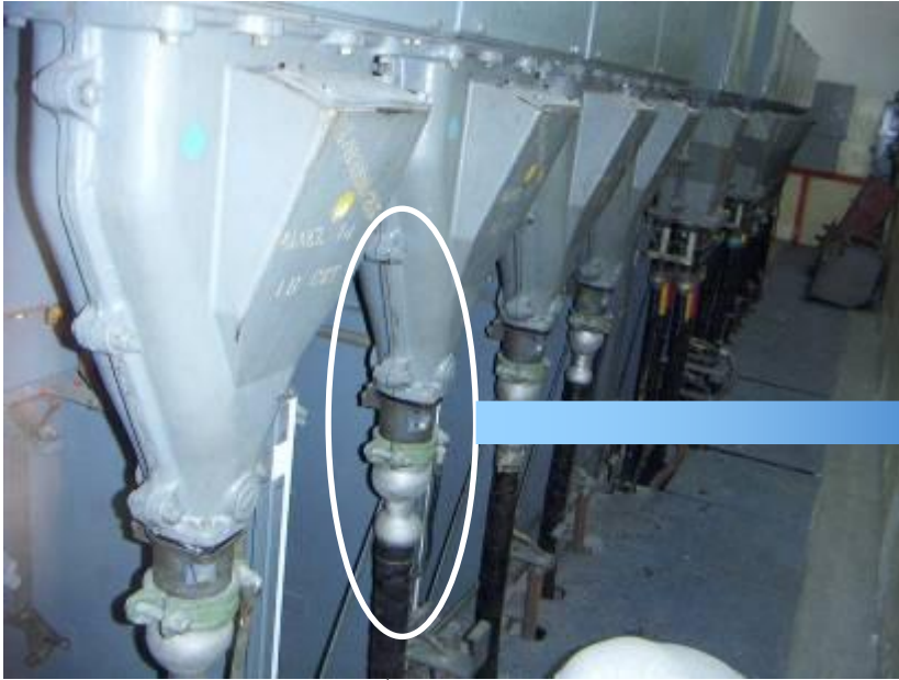
↑ 11kV three core cable
