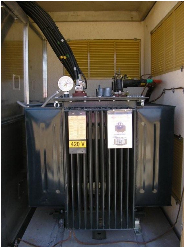
Transformer just after installation
